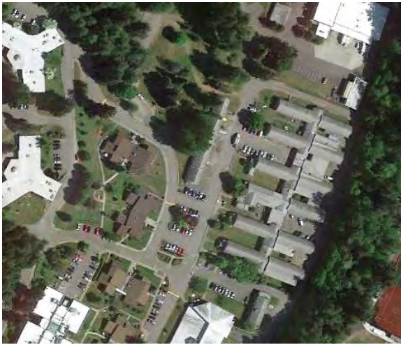
Figure 10 Aerial image of Area 1
