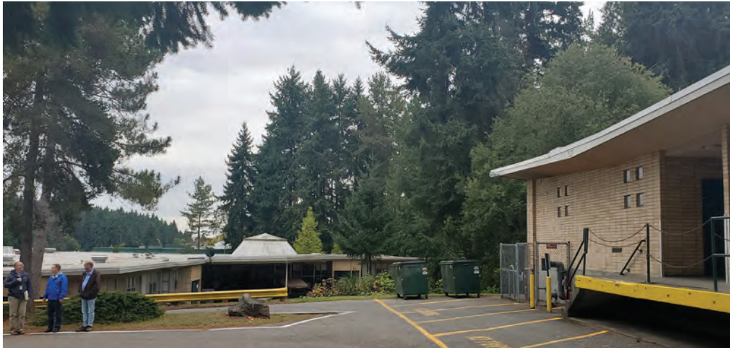
Building Area 1: North
