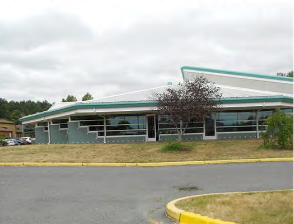
SOUTH SIDE OF CAFETERIA BUILDING
