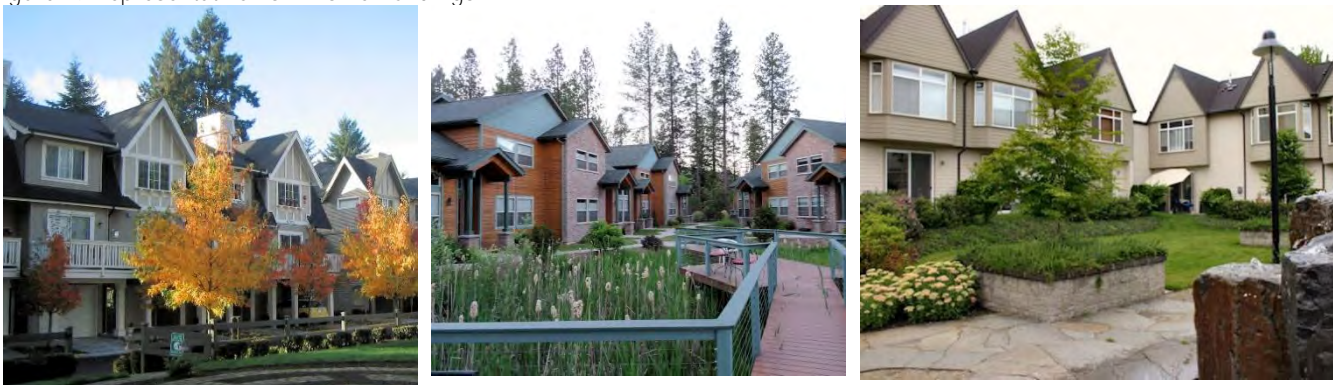
Figure 19 Representative Townhome Buildings
