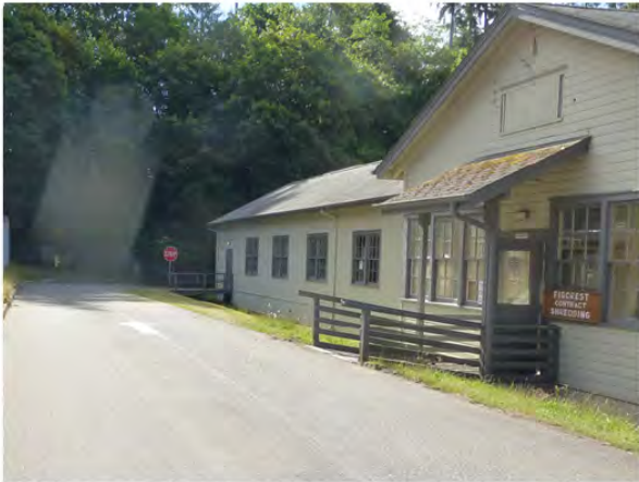
ATP BUILDING - WEST ROAD - PORTION OF HAMLIN CREEK IS PIPED DOWN ROAD
