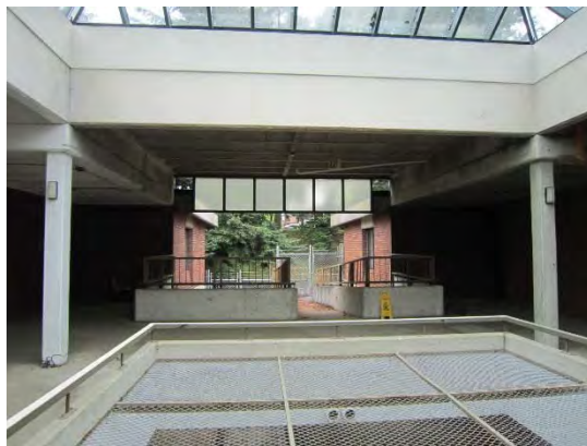
Photo 3 – Courtyard with Planter at Level 3
