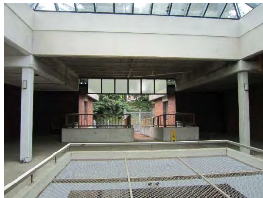
Photo 3 – Courtyard with Planter at Level 3
