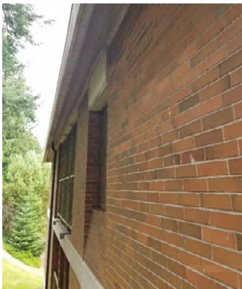
Exterior Wall at Roof Overhang
