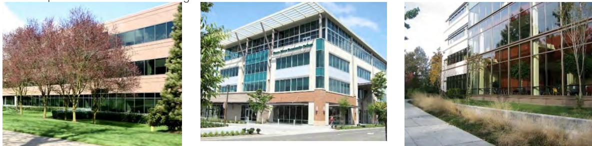
Figure 20 Representative office buildings
