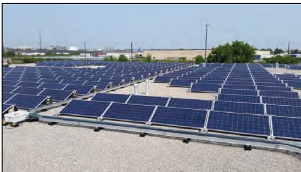
Figure 6: Ballasted racking installation system on flat roof
