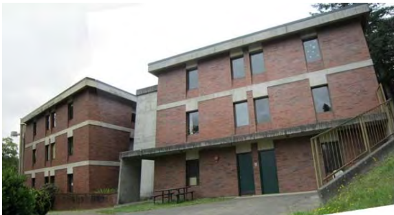
Photo 1 – East Elevation of Building
