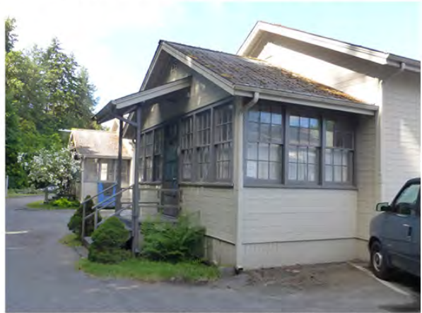
ATP BUILDING - WEST ROAD - PORTION OF HAMLIN CREEK IS PIPED DOWN ROAD
