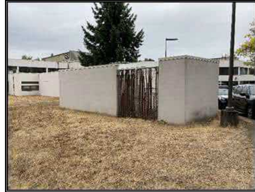
East Campus Well House
