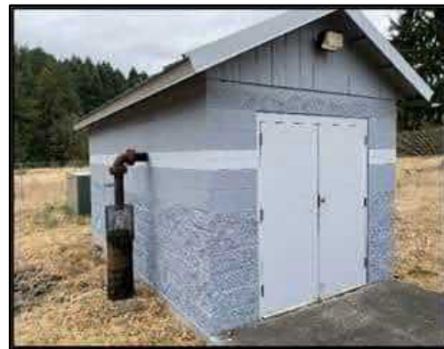
Farm Well House
